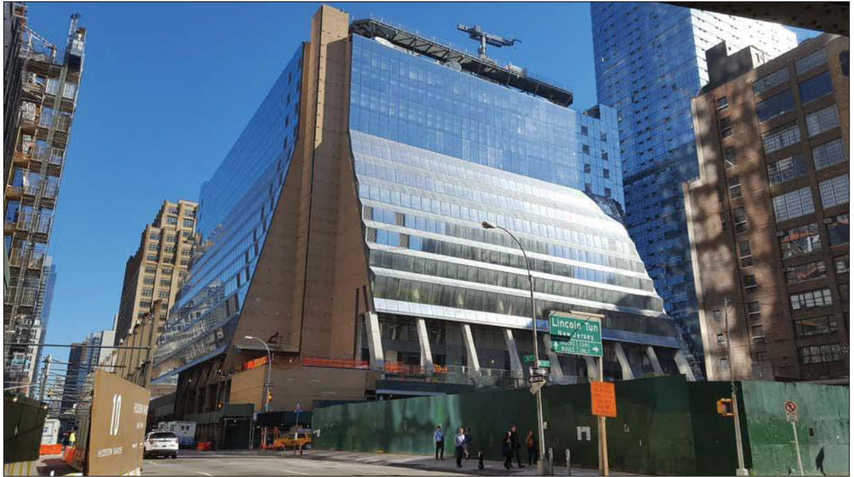
View northeast on Tenth Avenue, including the Lerner Building on the east side of Tenth Avenue between West 31st and West 33rd Streets. 2
