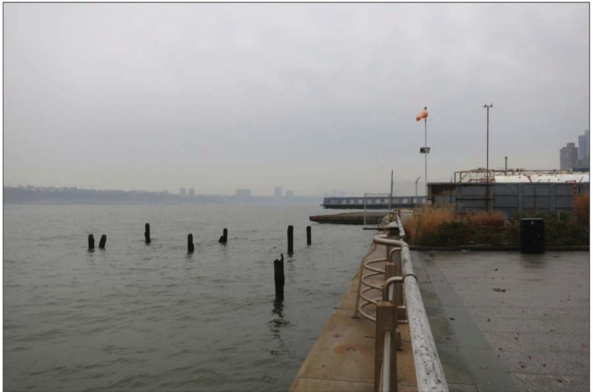
View north at the the Hudson River bulkhead in the location where the new tunnel would cross through the bulkhead and where ground improvements would also be needed to construct the tunnel. 4
