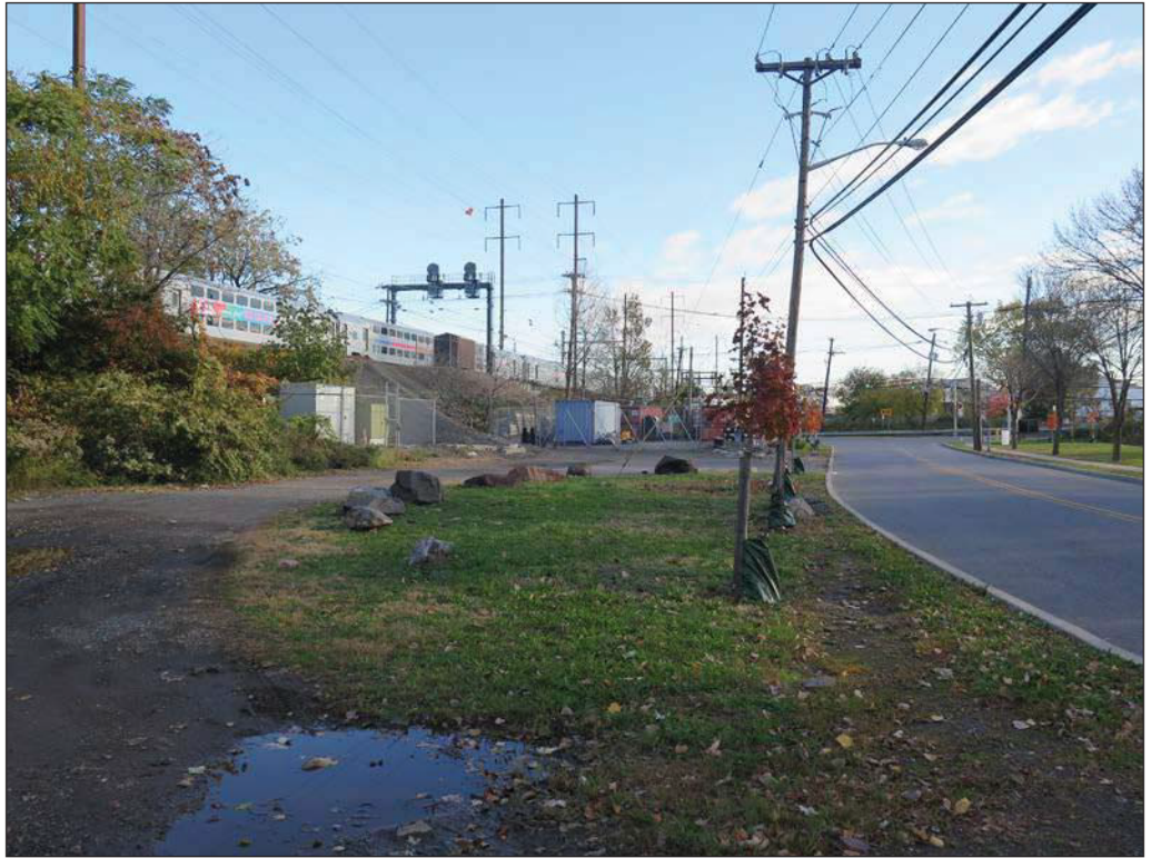
View northeast on Penhorn Avenue, west of Secaucus Road, of the existing NEC and location of a proposed entry to the access road. 4
