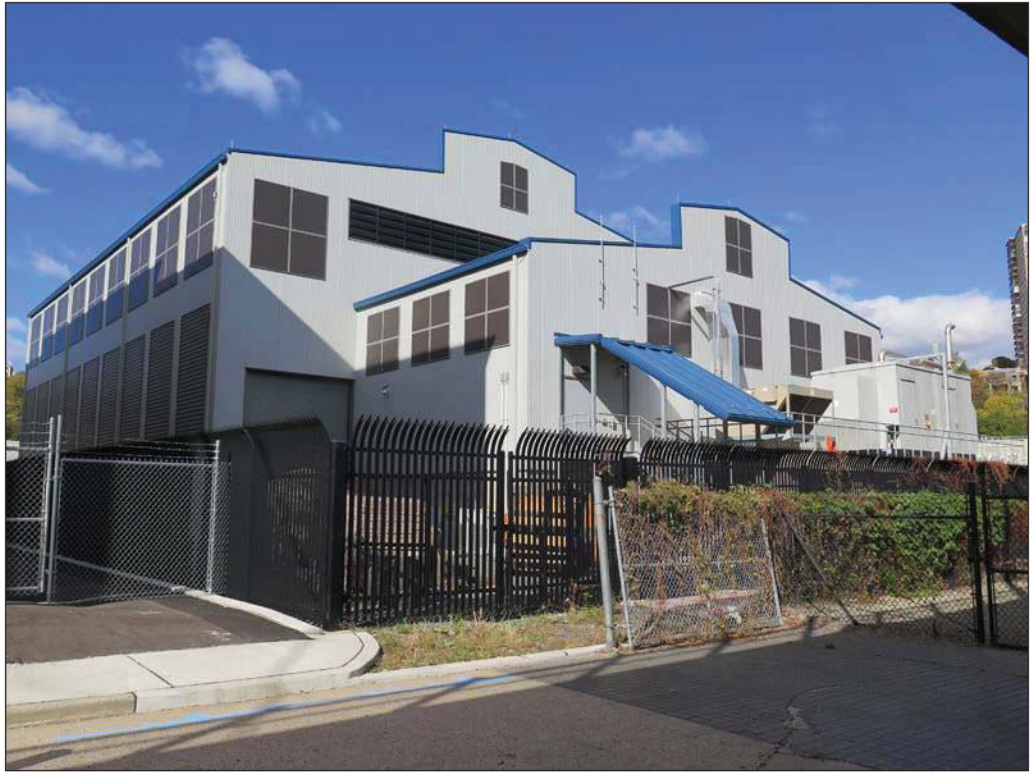
View northwest of the location of potential ground improvements west of Willow Avenue. 10
