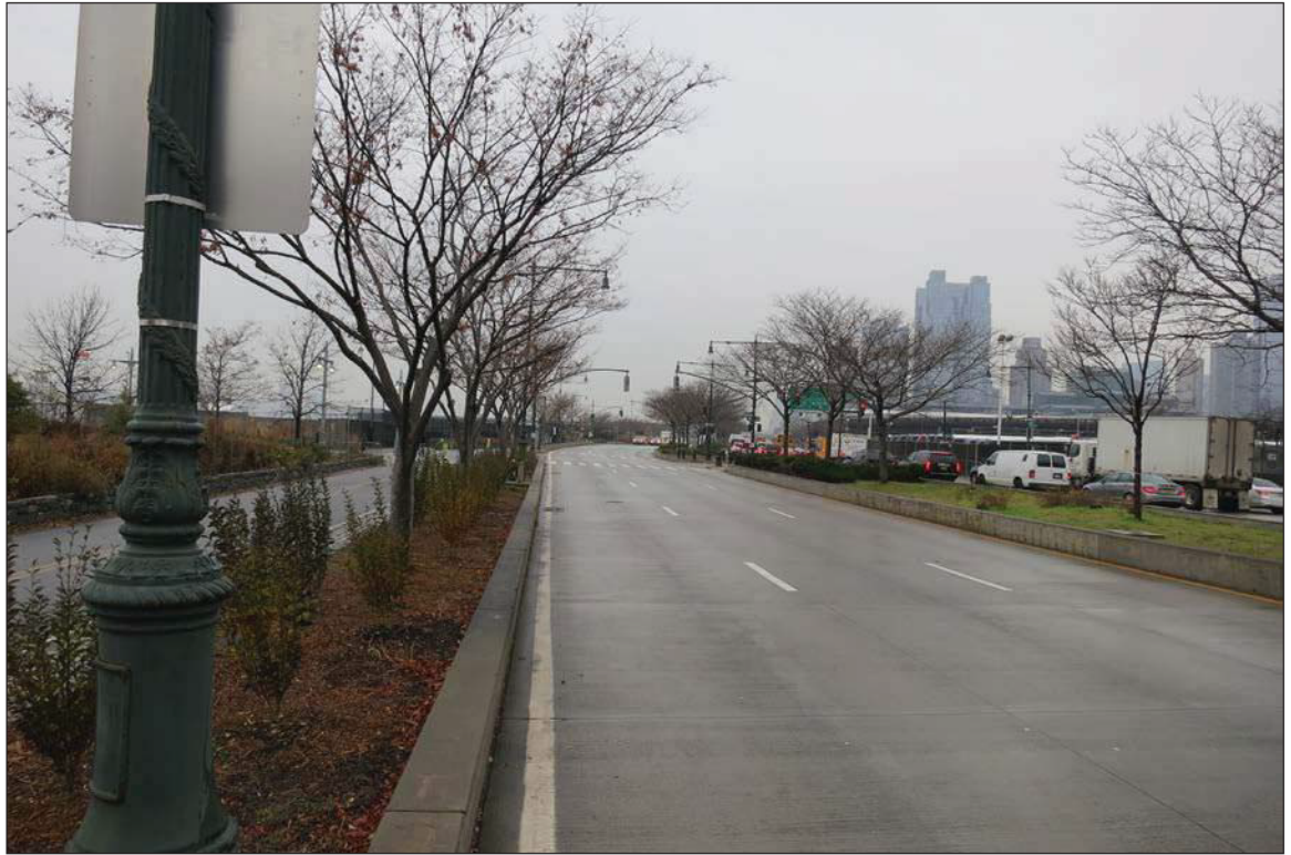
View north on Route 9A/Twelfth Avenue towards the location where ground improvements would occur to construct the new tunnel. The location of the proposed ventilation shaft site and fan plant is on the right.
